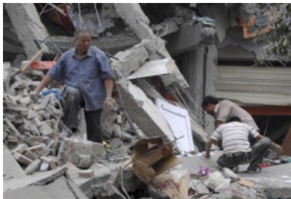
Slika 7. Reševanje iz ruševin je bilo zelo zahtevno in marsikje onemogočeno; prvič zaradi oteženega ali nemožnega dostopa zaradi porušeni cest in drugih dovoznih poti in drugič zaradi porušitev, saj so bili številni objekti v celoti porušeni v sistemu »palačink« (vsa nadstropja se porušijo in pod seboj stisnejo vse) Figure 7. Rescuing from the ruins was very pretentious and in many places impossible; first because of the difficult or impossible access due to ruined roads and other access ways and second because of ruins, because many buildings were completely ruined in a 'pancake' system (all floors collapse and press everything under)
