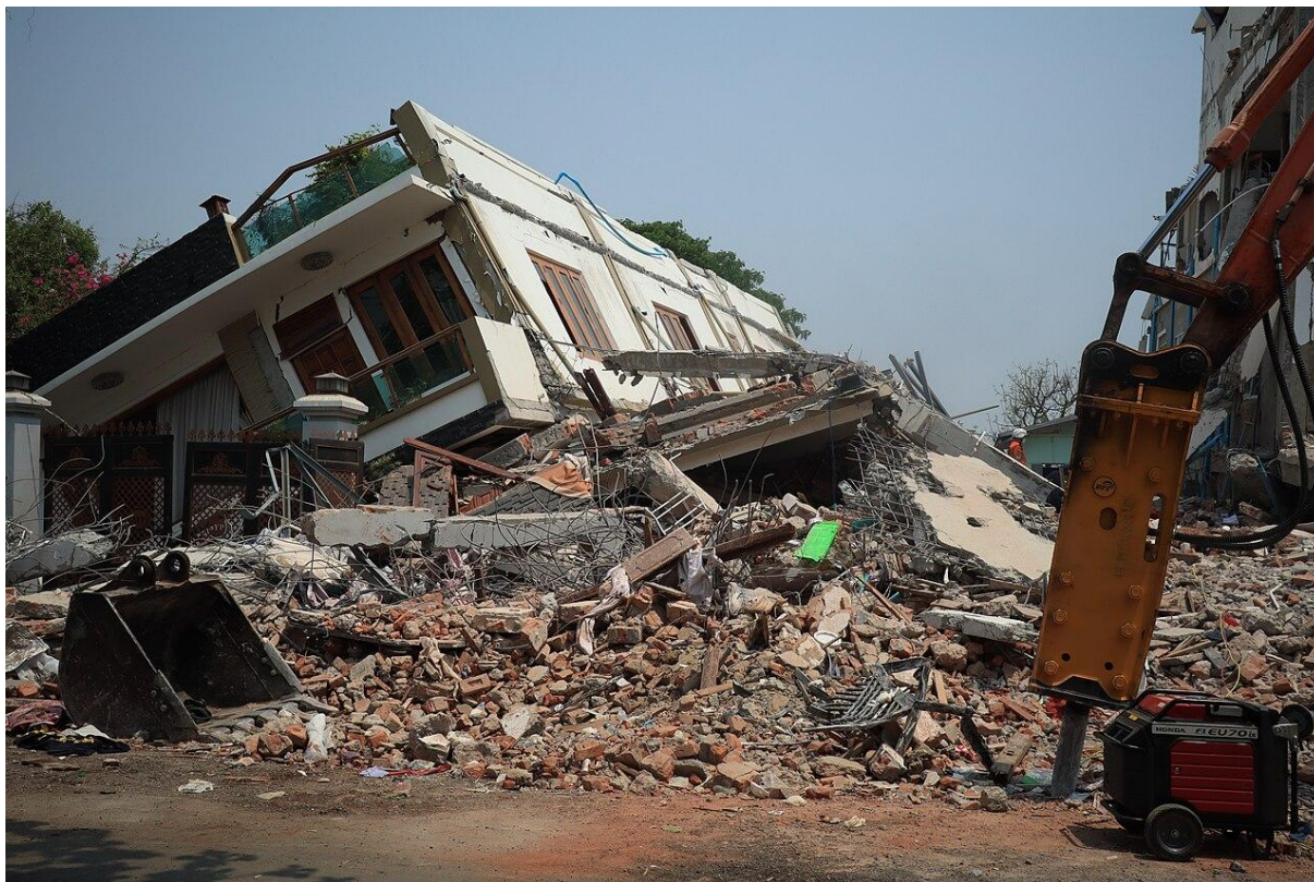
Slika 7. Porušena stavba v Mandalaju (vir: https://en.wikipedia.org/wiki/2025_Myanmar_earthquake#cite_note-31 )
