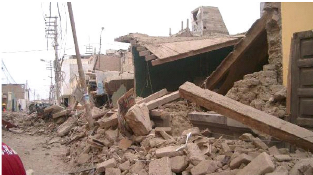
Slika 2. Značilna porušitev hiš zgrajenih iz na zraku sušene opeke. Tovrstne poškodbe so prevladovali v krajih Pisco, Ica in Chincha Alta Figure 2. Typical demolition of houses built of the air-dried brick. Suchlike ruins predominated in Pisco, Ica in Chincha Alta
